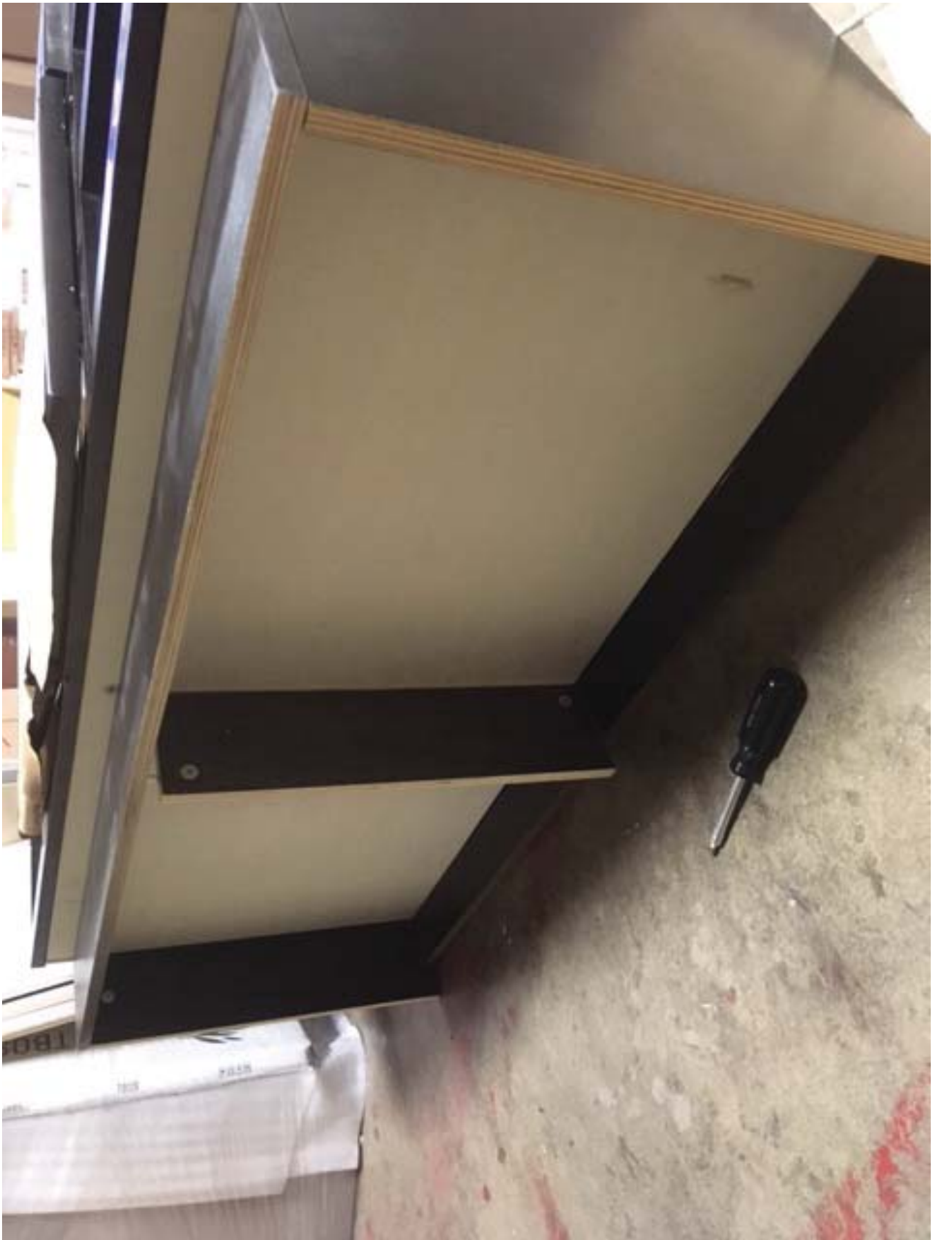
Install kick board.
